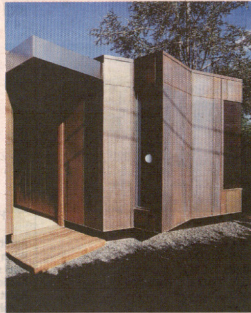
Pre-weathered copper sheets are used on external walls of the extension. PICTURE: MEINPHOTO
